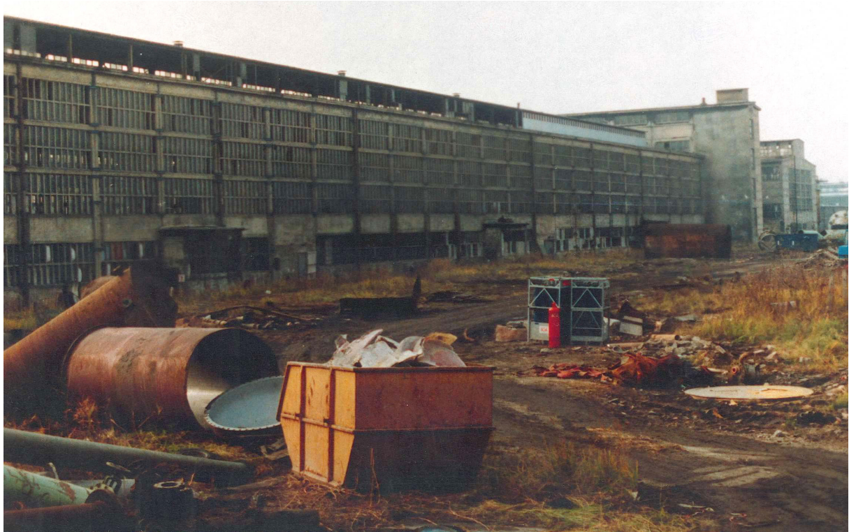
Figure 4.1: Chlor-alkali production facility L 66 at BSL Werk Schkopau before demolition was started
